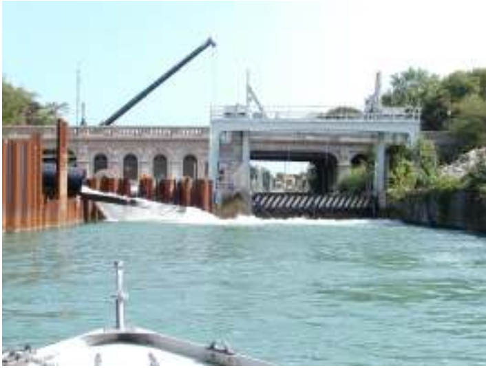
North Branch of Chicago River lock at Wilmette, Illinois, looking east toward Wilmette Harbor. In times of extremely heavy rains, these gates are opened to relieve flooding. Courtesy: Chicago Sun-Times blog.
